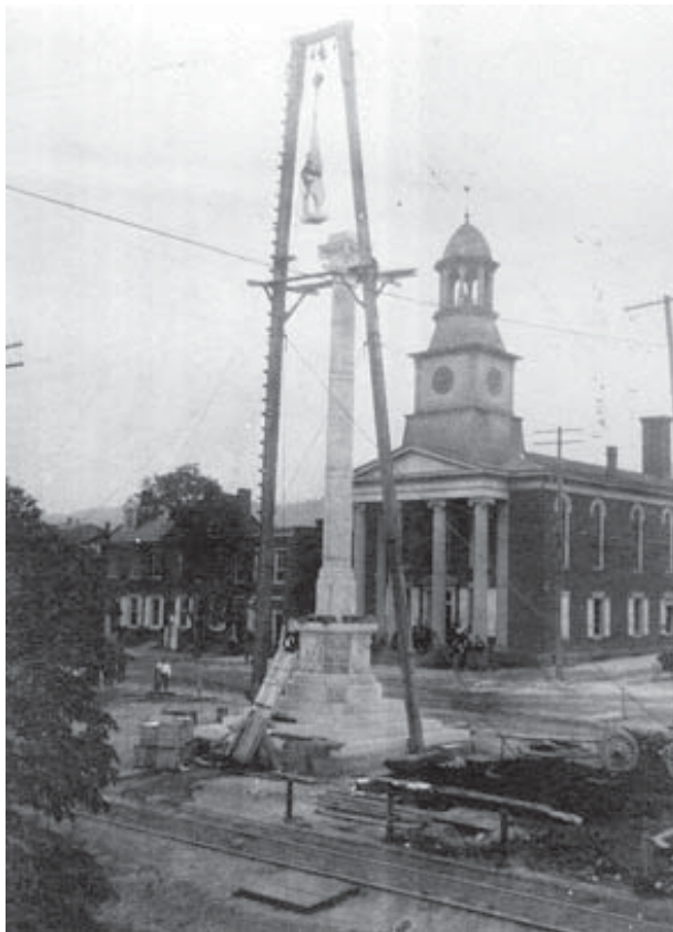
Erecting the Soldiers' and Sailors' Monument
