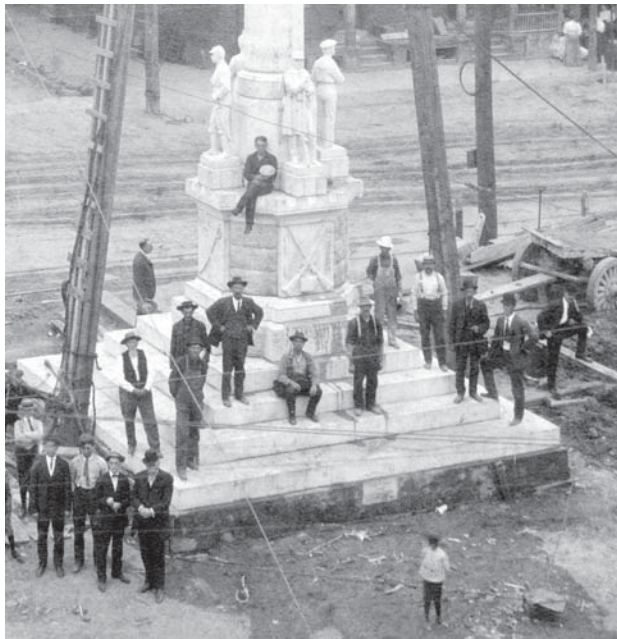
Work completed June, 1906 - Workmen from Lewistown contractor D. R. Stratford and men from the Moore Brothers and Brault Company, Granite Manufacturers from Barre, Vermont, take a much deserved break after setting the finishing touches on the Soldiers' & Sailors' Monument. At the base of the monument, is a special stone which came from the tomb of Abraham Lincoln. It can be seen as a white rectangle in the base directly behind the boy standing in front.
